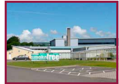
Figure 5.35 Front entrance to the NW Regional College
