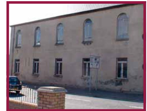
Figure 5.52 Existing vacant building along Connell Street
