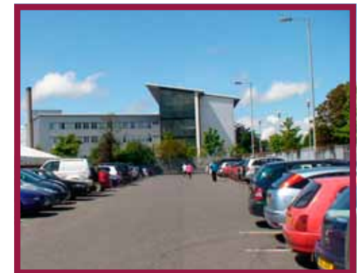
Figure 5.36 Rear entrance to the NW Regional College
