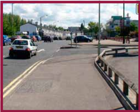
Figure 5.24 Existing access point to Connell Street car park
