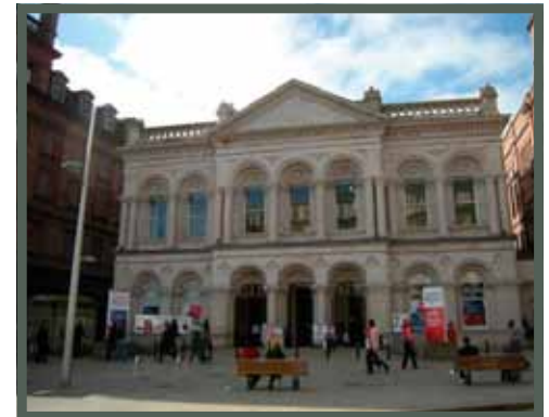
Figure 6.18 Example of a sensitive restoration in a town centre
