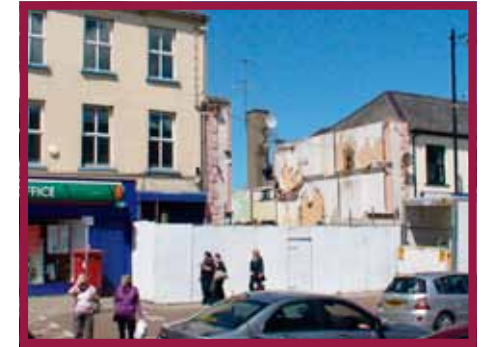
Figure 5.28 Existing gap site along Main Street
