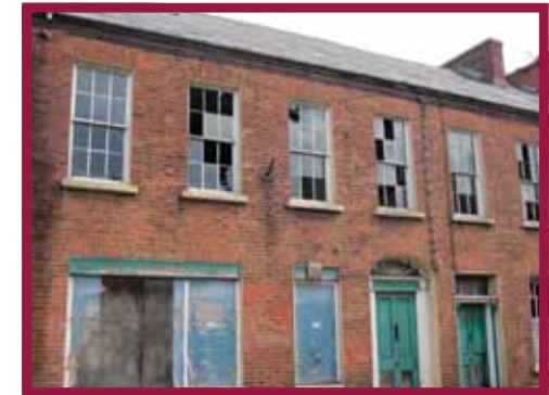
Figure 5.49 Derelict listed buildings fronting Linenhall Street
