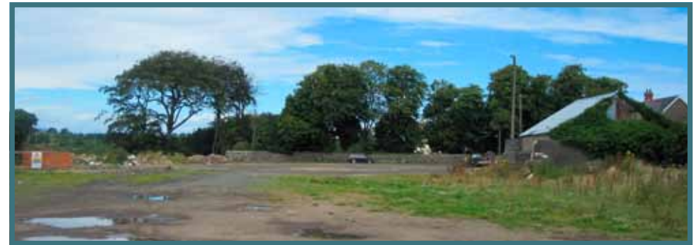
Figure 2.23 The Market Yard from Catherine Street
