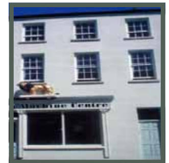
Figure 6.33 Example of a high quality shop front at ground floor
