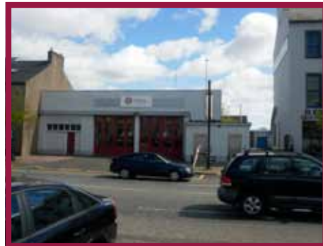
Figure 5.59 Entrance to former Limavady Printing Company site
