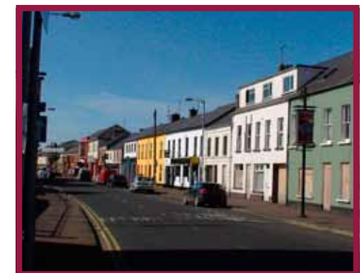
Figure 5.53 Existing vacant buildings fronting Irish Green St
