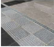
Tactile paving points: To match with main footpath material. Sympathetic to historic character of the town.
