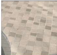
Parking/ Shared Surface: Stone setts Granite bullnose kerbs - sawn all sides, 20mm bullnose granite drop kerb
