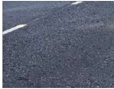
Main Road: Asphalt with chipping
