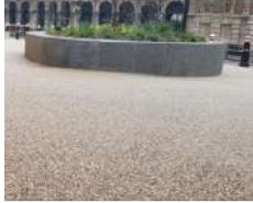
Main Diamond area - hard wearing for traders / events: Exposed aggregate concrete
