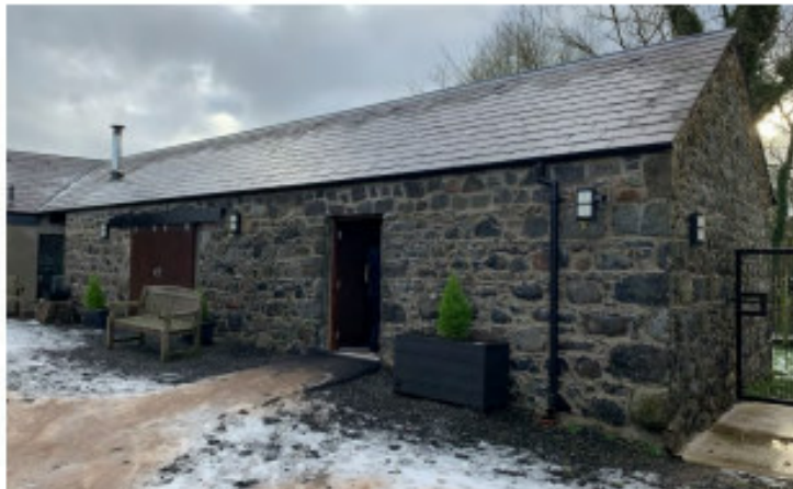
III 03 Cloughmills Old Mill building with flooding mitigation built in to the building.
