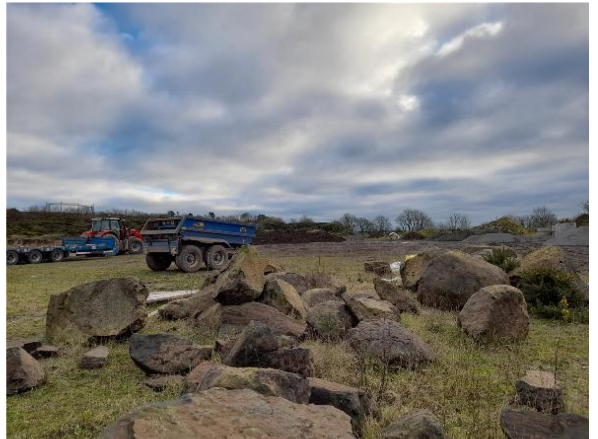
View from upper site looking south
