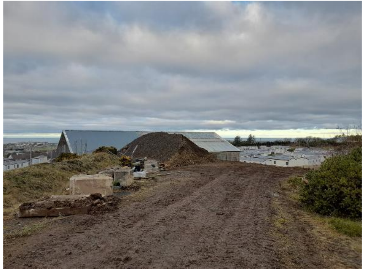
View from upper site at location of proposed Units 23 – 26 looking north
