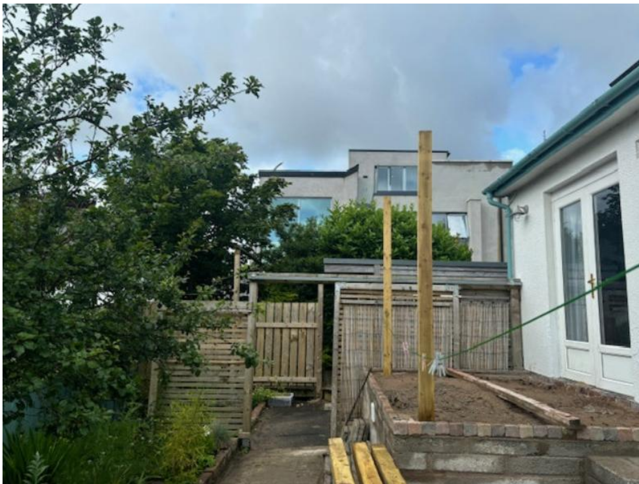
View from No 8 Cedar Drive
