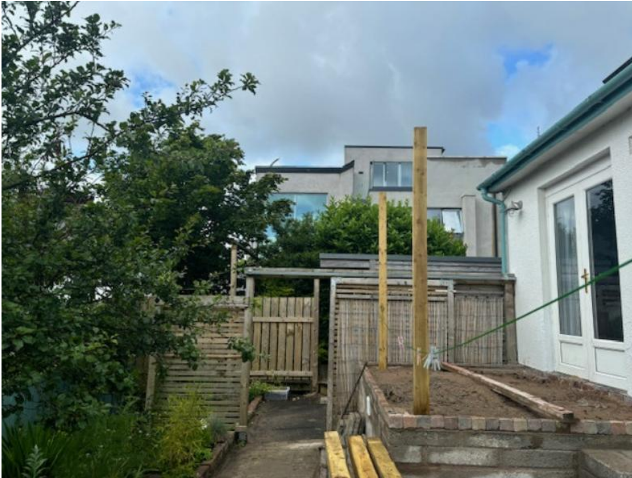
View from No 8 Cedar Drive
