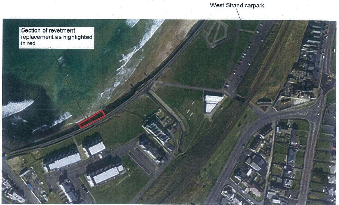
AERIAL PHOTOGRAPH INDICATING LOCATION OF WORKS
