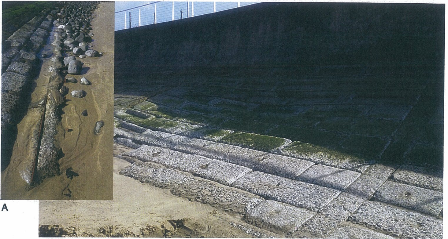
PHOTOGRAPH A & B indicating sections of pre-cast concrete revetment units having collapsed, with deterioration of sheet piling and cast in-situ concrete along bottom section of pier.
