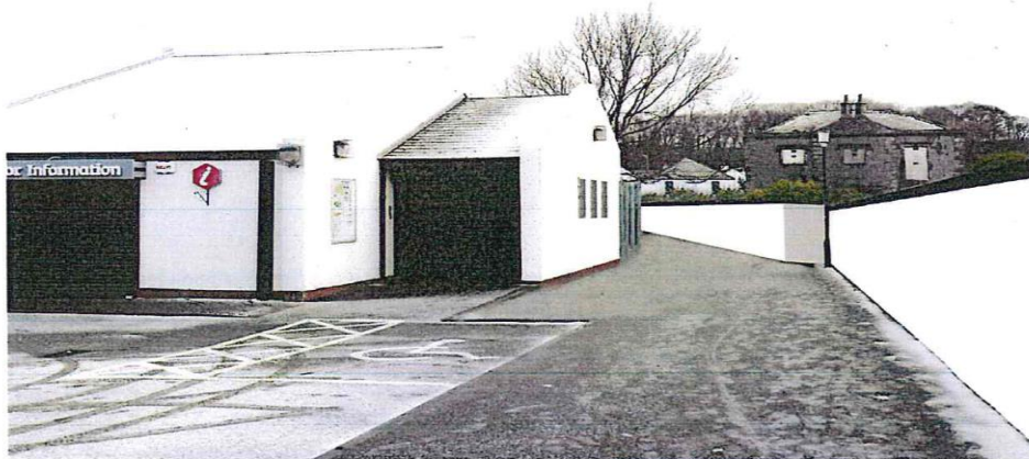
view after removal and re-alignment, plus wall painted prior to artwork installation.
