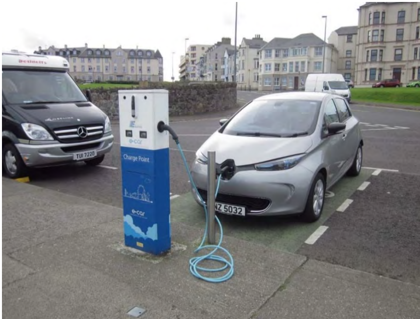
Electric car parking space and charge point at Bath Road, Portrush.
