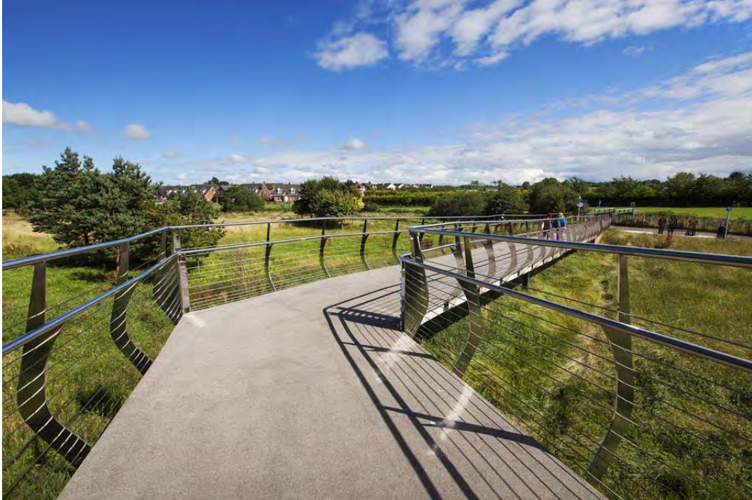
The cycle/footbridge's connection with the Riverside Park, with residential areas beyond.
