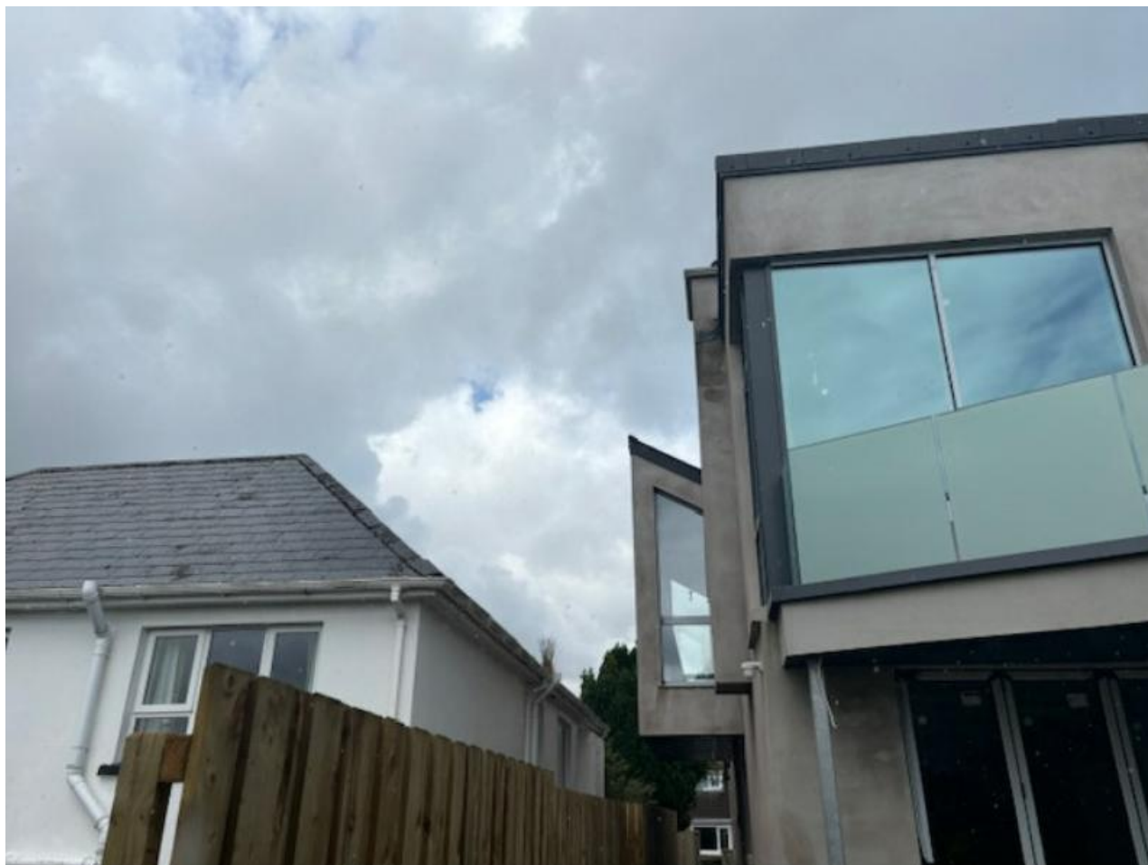
Rear elevation and No 6 Cedar Avenue
