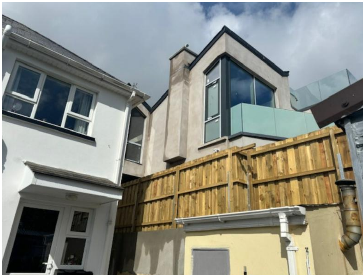
View from No 6 Cedar Avenue
