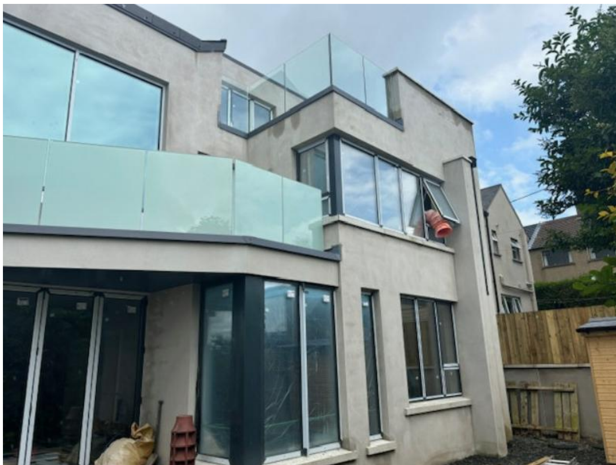
Rear Elevation and No 10 Cedar Avenue
