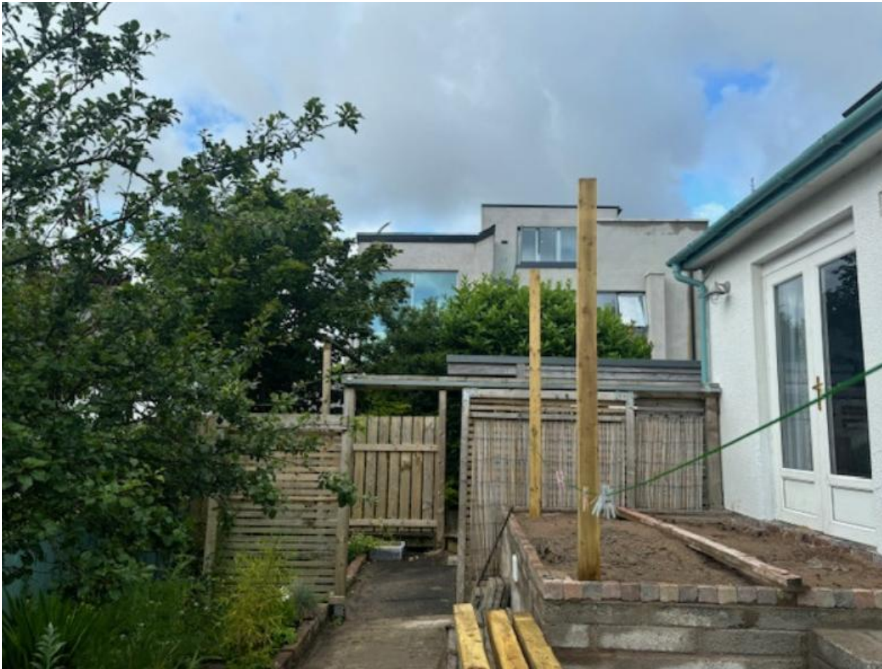
View from No 8 Cedar Drive
