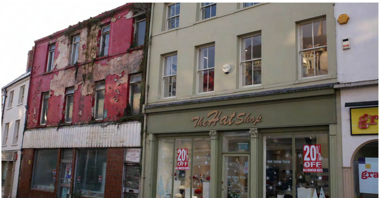
Adjacent properties on Bridge Street before and after refurbishment
