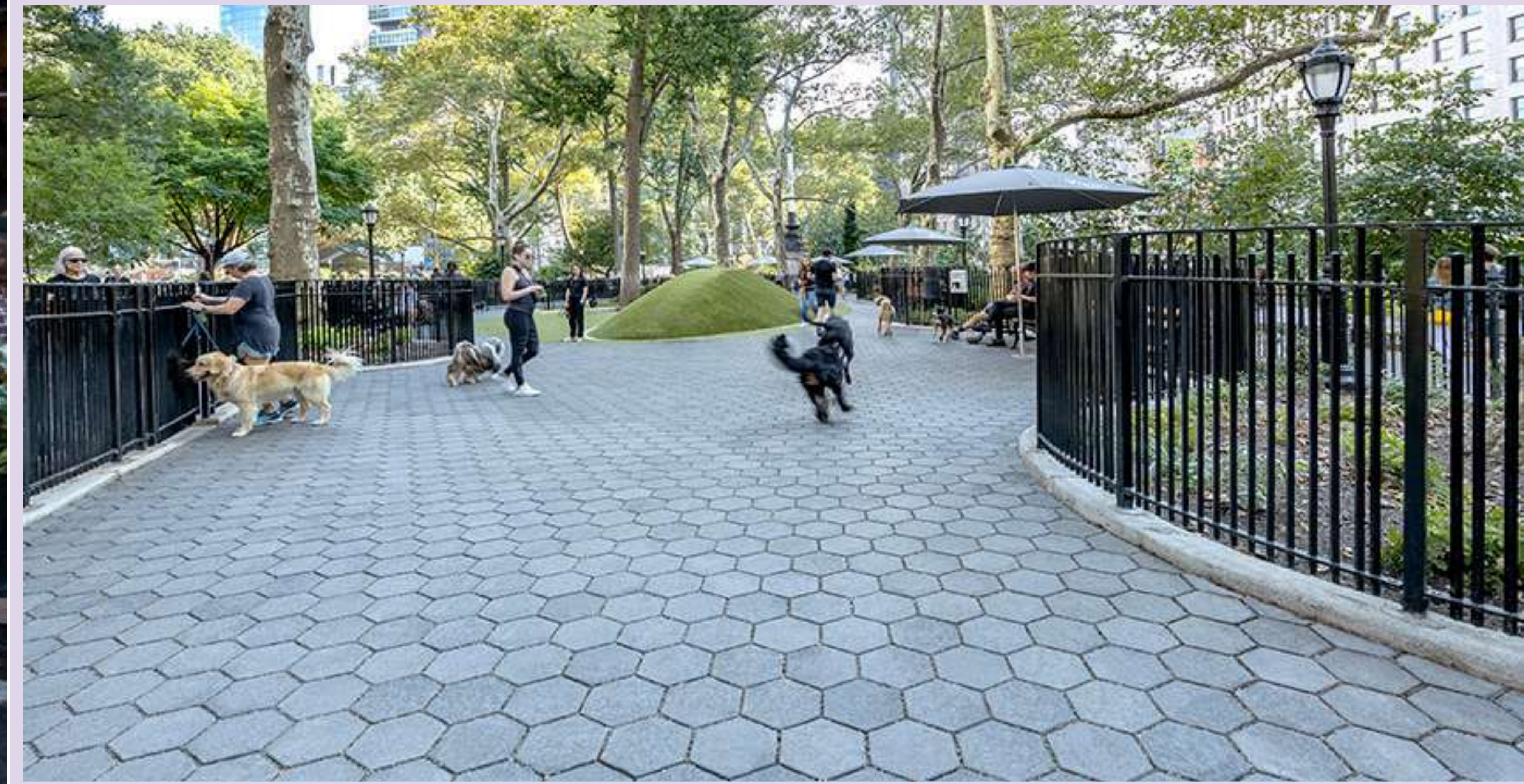
Manhattan - Concrete Hexagonal, Permeable and climate positive paving.
