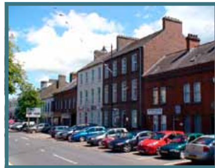
Figure 2.8 Georgian buildings on Main Street
