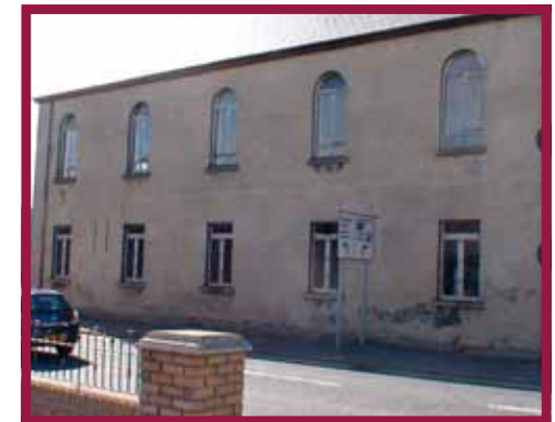
Figure 5.52 Existing vacant building along Connell Street
