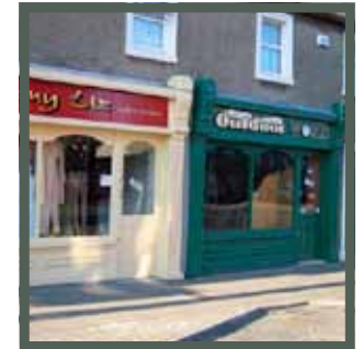
Figure 6.31 Example of sensitively restored shop front
