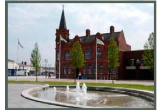
Figure 6.19 Example of high quality setting for a listed building
