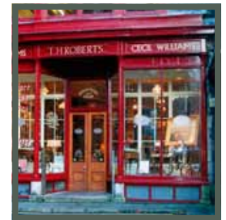
Figure 6.32 Example of sensitively restored shop front
