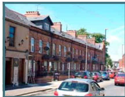
Figure 2.9 Historic terrace on Linenhall Street
