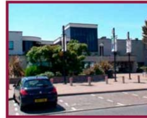
Figure 5.30 Forecourt of Limavady Borough Council offices
