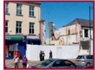
Figure 5.28 Existing gap site along Main Street
