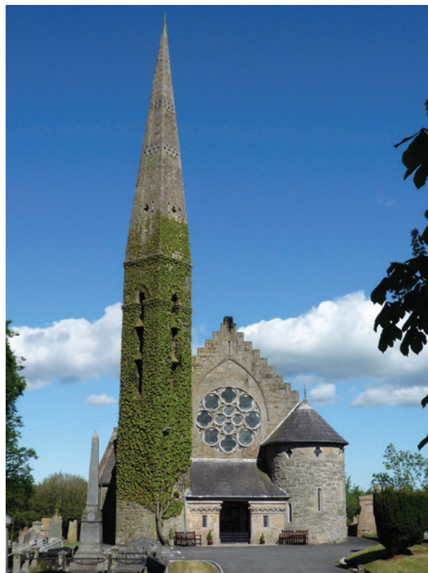
Christ Church of Ireland, Derriagh Road, Magheralave, Lisburn, Co. Antrim
